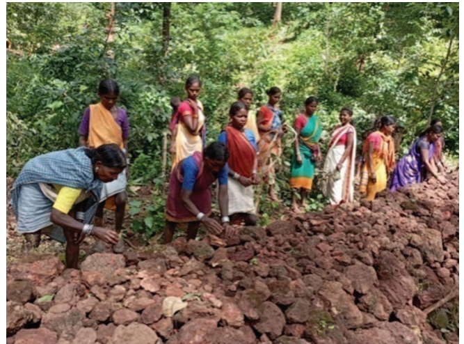
FIGURE 2 Bolder check-dam construction
